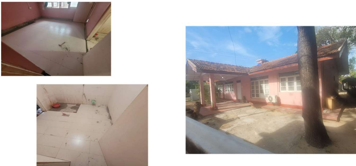
Renovation of old MS quarters building at DGH Mannar
