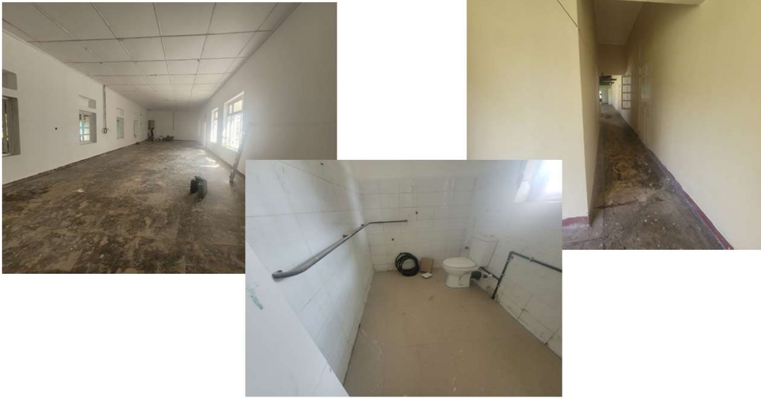
Renovation of old ward 3 at DGH Mannar
