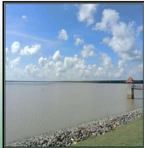
Sluice and riprap
