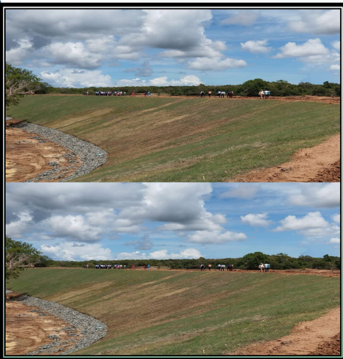
Completed Bund and toe drain
