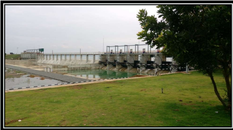
Completed New radial Gates on LB side
