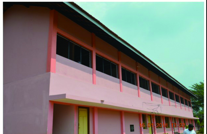
26 .Construction of Classroom Building (Upper floor) 110x25x2 - Stage 02 at Vu/Poonthoddam M.V
