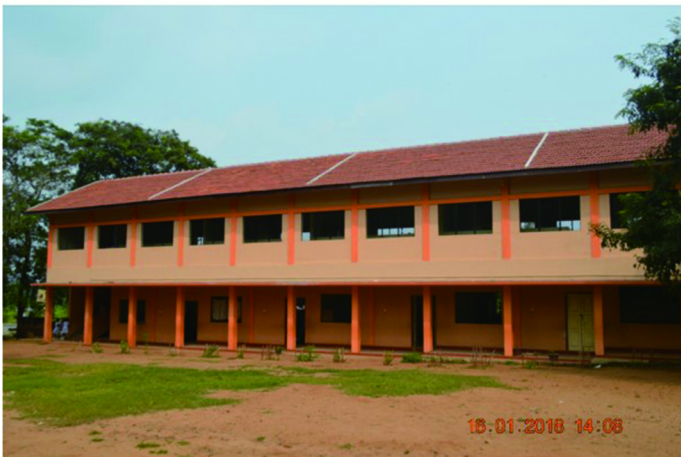
25. Construction of Classroom Building 110X25X2 (Upper floor) - Stage 02 at Vu/Bogaswewa GSMS
